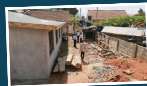
Commencement of animal house renovation works
