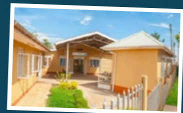
Completion of renovation works for the MLI office block + clinic
