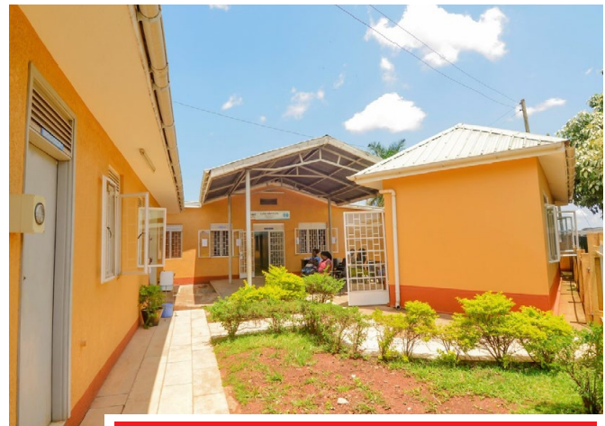
MLI Central block before renovation (left) and after renovation (right).
